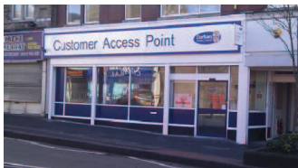
Customer Access Point Consett
