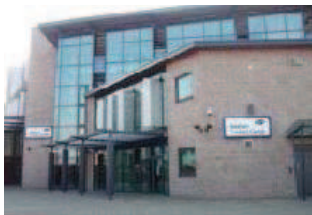
Customer Access Point Seaham
