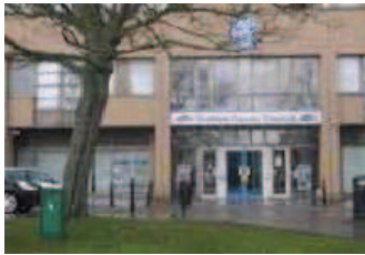
Customer Access Point Crook
