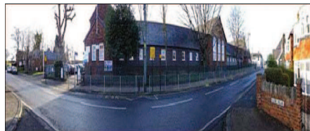
West Cornforth Primary School
