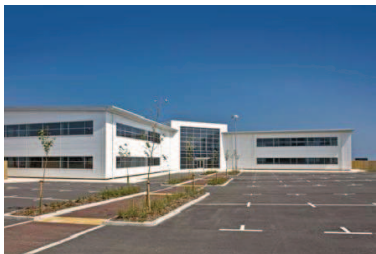
Office Accommodation, Spectrum Business Centre, Peterlee
